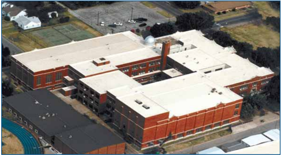
Photo 3 – According to roofing contractor Rod Heitfield, owner and president of Heritage Roofing Systems in Enid, Oklahoma, energy savings from the cool roofs installed in several other district schools were so great that they virtually paid for the entire 81,803-square-foot PVC cool roofing system protecting Enid High School. (Photo courtesy of Duro-Last Roofing, Inc.)
