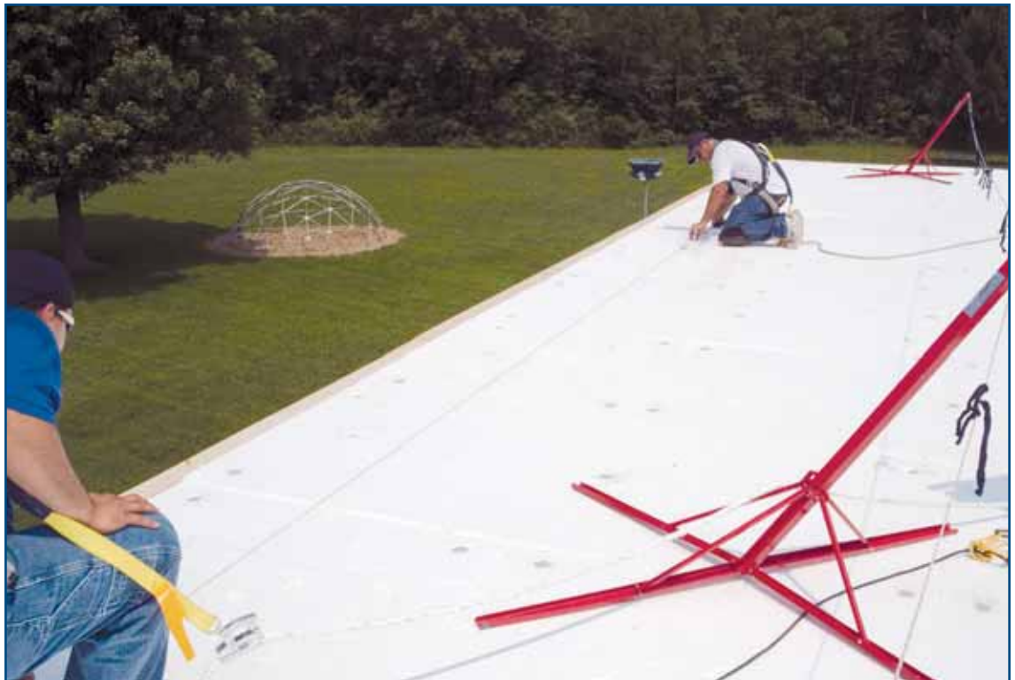
Photo 5 – Custom, pre-fabricated, single-ply roofing systems are precisely measured in advance to fit each roofing job. This reduces material waste, labor requirements and installation time, and minimizes the risk of human error by performing most of the seaming in the factory under controlled conditions. (Photo courtesy of Duro-Last Roofing, Inc.)
