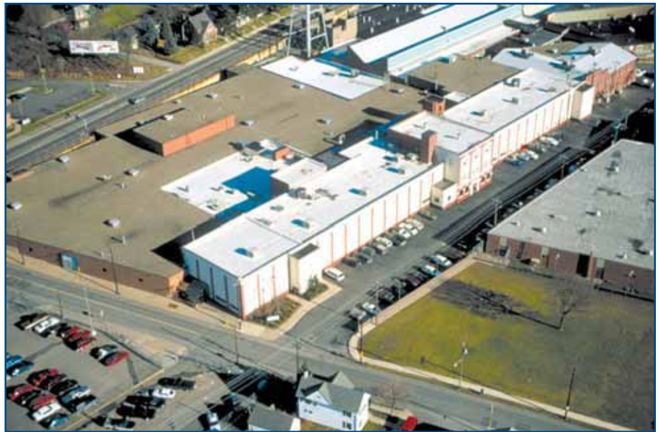
Photo 6 – High-performance roofing systems moderate indoor temperatures, even in buildings that are not fully air-conditioned at all times, such as the Textron manufacturing facility in Williamsport, Pennsylvania. Various studies have shown a direct relationship among thermal comfort, overall mental concentration, and manual work rates. (Photo courtesy of Duro-Last Roofing, Inc.)
