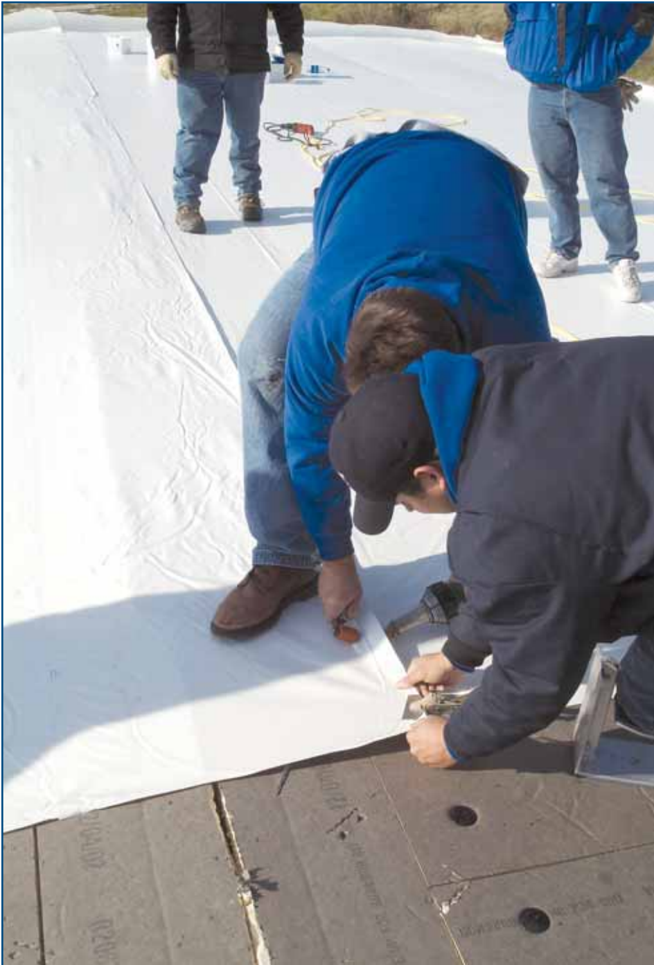
Photo 1 – Thermal insulation is a crucial part of HPR systems, reducing heat loss through convection in winter and controlling heat gain through conduction in the summer. Since cool roofing surfaces are significantly cooler than black surfaces on hot days, the underlying insulation can be 25 to 50 percent more effective at resisting thermal conductivity under summer heat loads. (Photo courtesy of Duro-Last Roofing, Inc.)
