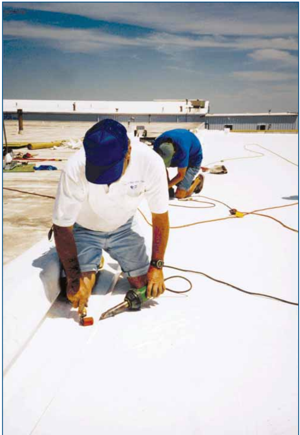
Photo 2 – By the late 1990s, cool roofing was the “hottest” trend in commercial roofing, and white thermoplastic single-plies began a sustained run as the fastest-growing category of commercial roofing systems. (Photo courtesy of Duro-Last Roofing, Inc.)
